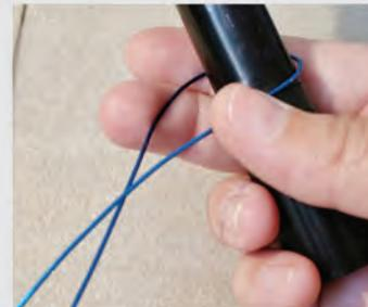
2. Wrap the wire around the marker 3 times, making sure not to cross it over. The loops should sit next to each other.
